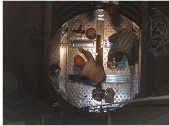
Figures -7 & 8 Field Installation of ADV ® -MP Trays
