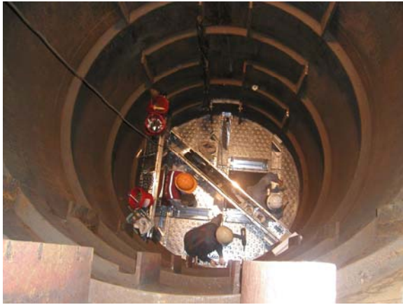
Figures -7 & 8 Field Installation of ADV ® -MP Trays
